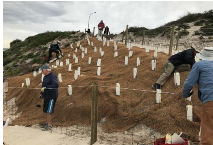
In winter 2021, Cambridge Coastcare members and volunteers planted alongside a new path which was constructed to direct foot traffic and minimise the dune erosion and vegetation destruction caused by people climbing up and down the steep dune. Photo – John Campbell.
