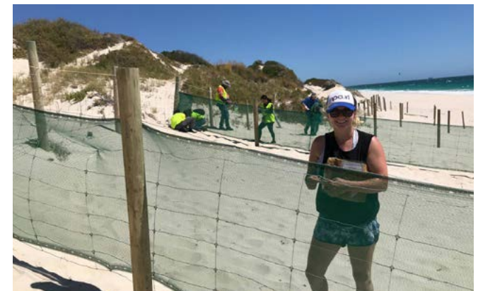
Completing work on drift fencing in 2017. Photo – John Campbell.
