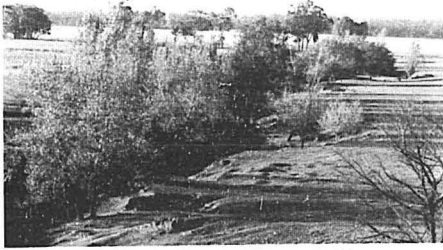
Trees alone are often insufficient to control streambank erosion.
