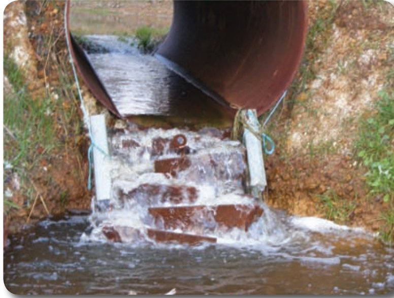
The western minnows can't get upstream? Remedy, build a fish ladder. Collie.
