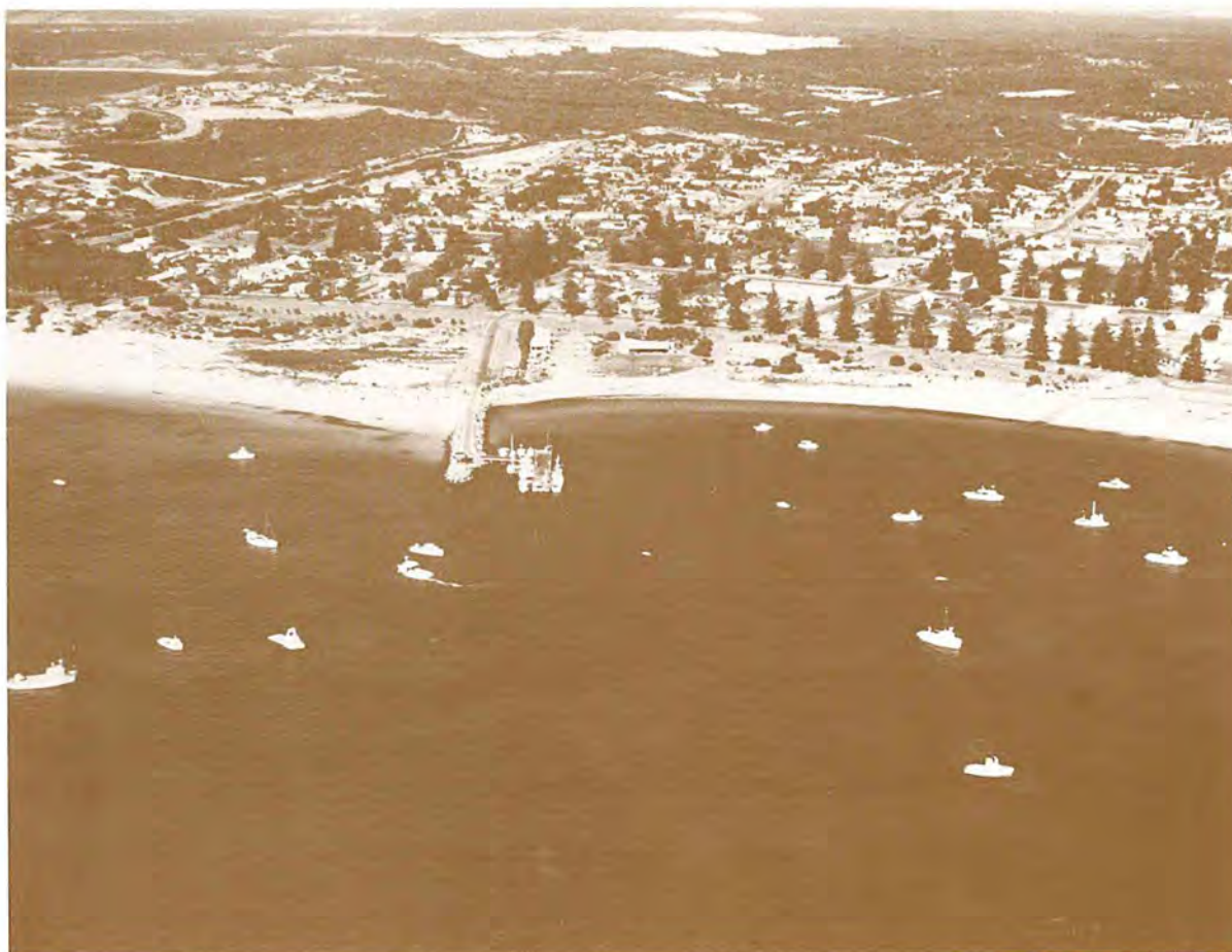
Photograph 7 Taylor Street Jetty, Esperance Bay Yacht Club, 20 tonne slipway and launching ramp.
