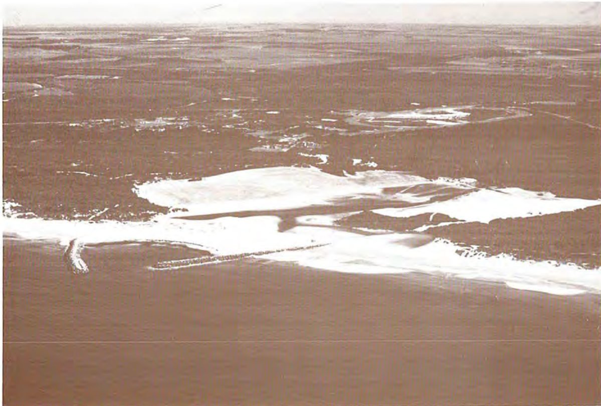
Photograph 4 Construction of the new boat harbour at Bandy Creek (October 1983).
