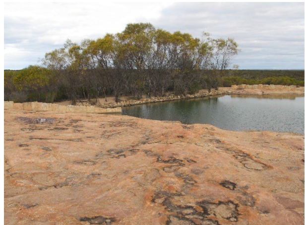
Acacia thicket growing along a dam wall sited on a large granite dome. Uplifted and cemented exfoliated granite slabs channel watershed into the dam
