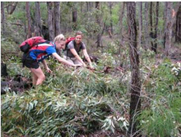
Mandy and Amy clearing storm damaged trees from their section of the Track
