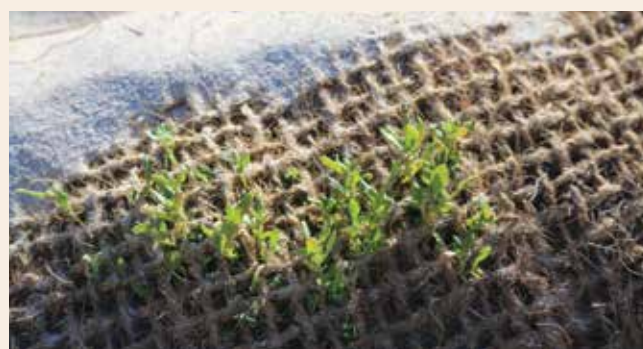
Top: Natural coconut fibre coir mesh matting installed at Five Fingers, Coral Bay, traps sand, seed and moisture. Above: Coir mesh matting allows for germination of native plant species.
