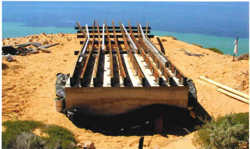
The lookout at Skip Jack Point under construction.
