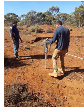
Fence line construction
