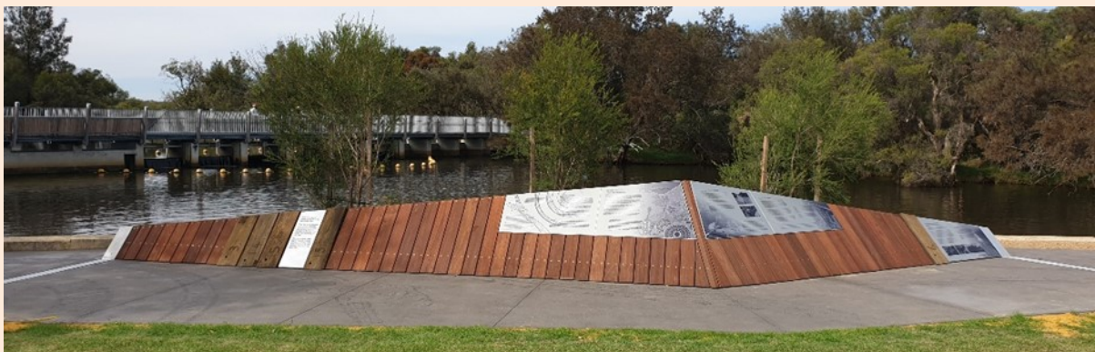
Completed Kent Street Weir node with interpretive signage. All photos—Sean Renner, Riverpark project officer.
