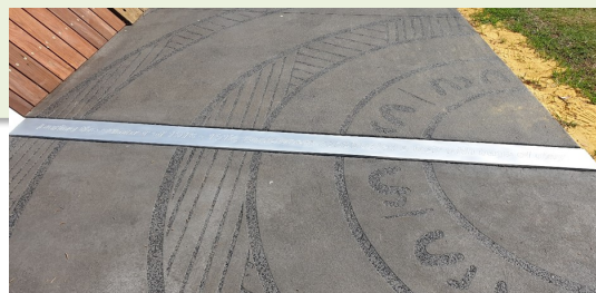
Local Whadjuk artist Justin Martin's design sandblasted on the new concrete path, with engraved text on aluminium strip. Photo – Sean Renner, Riverpark Project Officer, DBCA.
