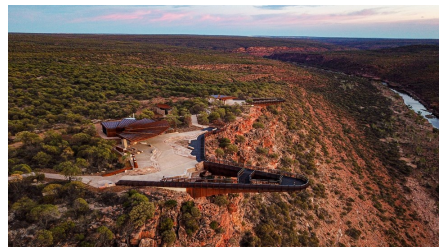
The Skywalk site overlooking the Murchison River
