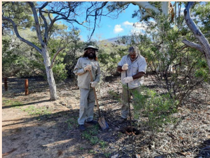
Burringurrah Rangers bollard replacement.
