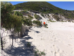
Installing dune fencing at Quarram - Photo by Chris Goodsell
