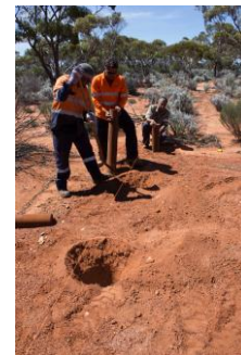
Bollard installation on campsite
