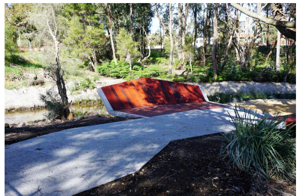
Decking installed at the Brentwood interpretation facility
