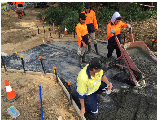
The trainees getting involved in pouring the concrete
