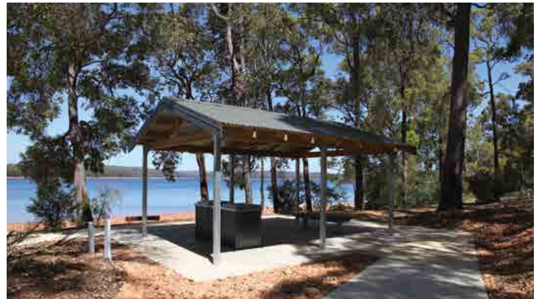
Sixty new camp sites were created and a day-use site upgraded at Potters Gorge campground in Wellington National Park. Photo – DBCA
