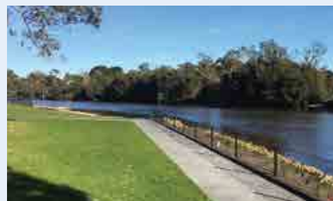
Improvements at Garvey Park included engineering and construction to stabilise the eroding riverbank. Photo – DBCA
