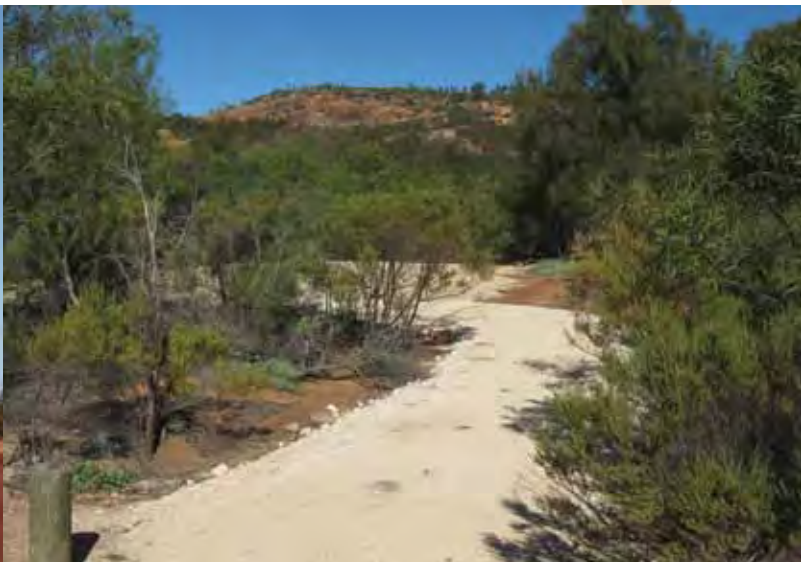
Access upgrades completed at Peak Charles National Park. Photo – Ian Hughes/DEC.
