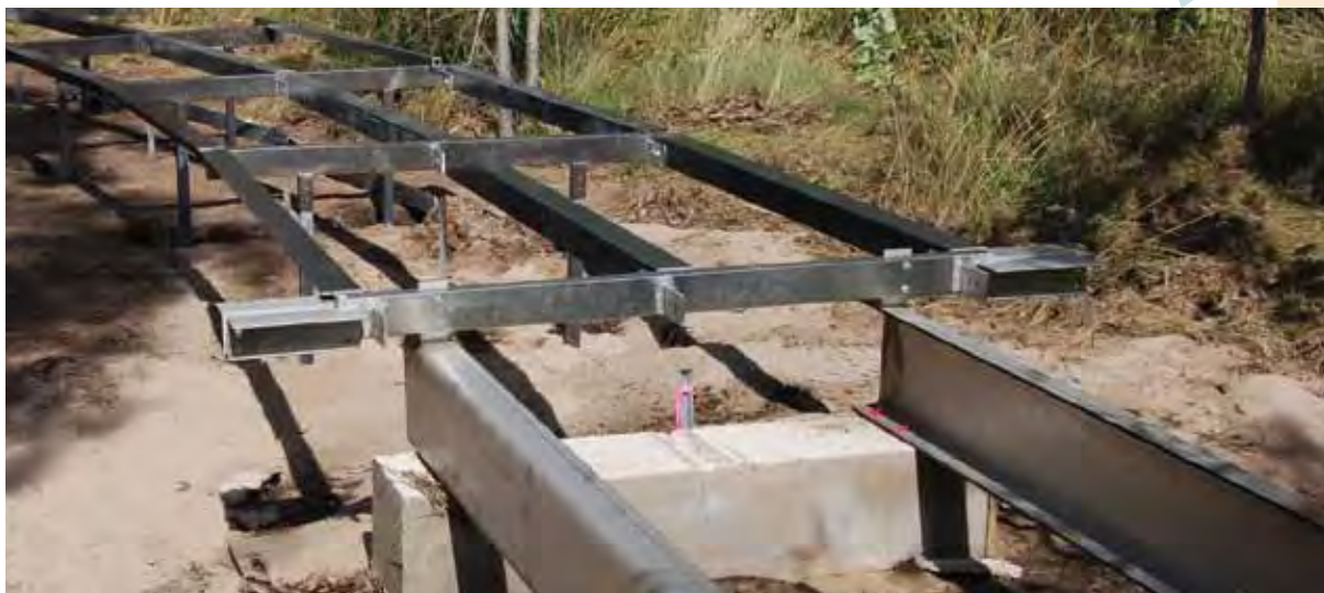
The boardwalk in Mirima National Park under construction.
