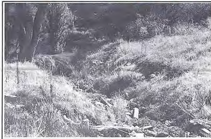
Southernwood Creek where it flows into the Southern River, Gosnells. Photo taken before work was carried out.
