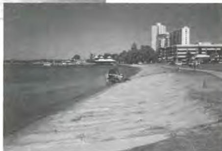
Above left: Walling at Sir James Mitchell Park in South Perth had broken away and left rubble on the shoreline and in the water. Centre: As part of Riverbank the collapsed walling was removed. Below: The area is now a beach that is more accessible to the community.
