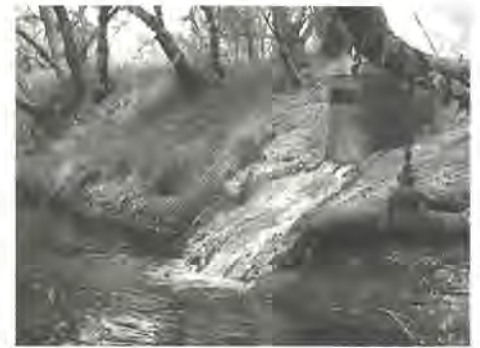
A release valve allowing scheme water to provide flows to the Canning River.
