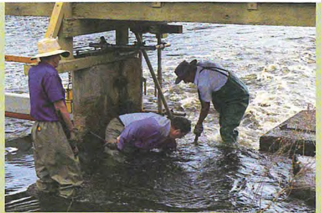
Weir boards are removed annually at the beginning of winter, and replaced at the beginning of summer to prevent habitat loss when the water level upstream can drop
