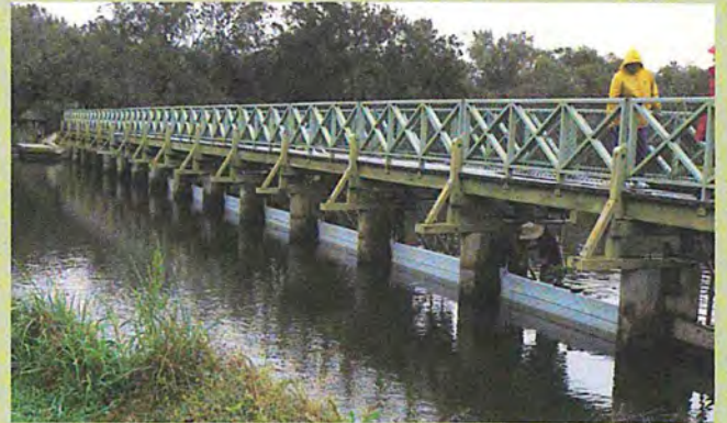
Weir boards are removed annually at the beginning of winter, and replaced at the beginning of summer to prevent habitat loss when the water level upstream can drop
