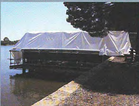
Above: A corroded section of the Ellam Street jetty in South Perth
