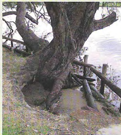
Eroded foreshore near Tranby House
