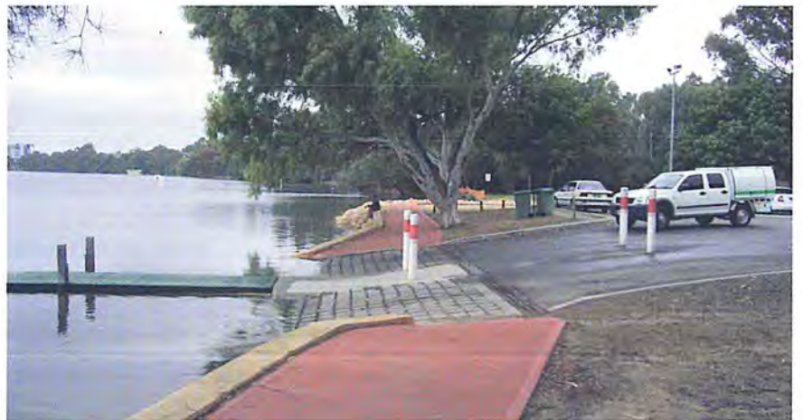
New limestone river wall and rock revetment in Belmont.
