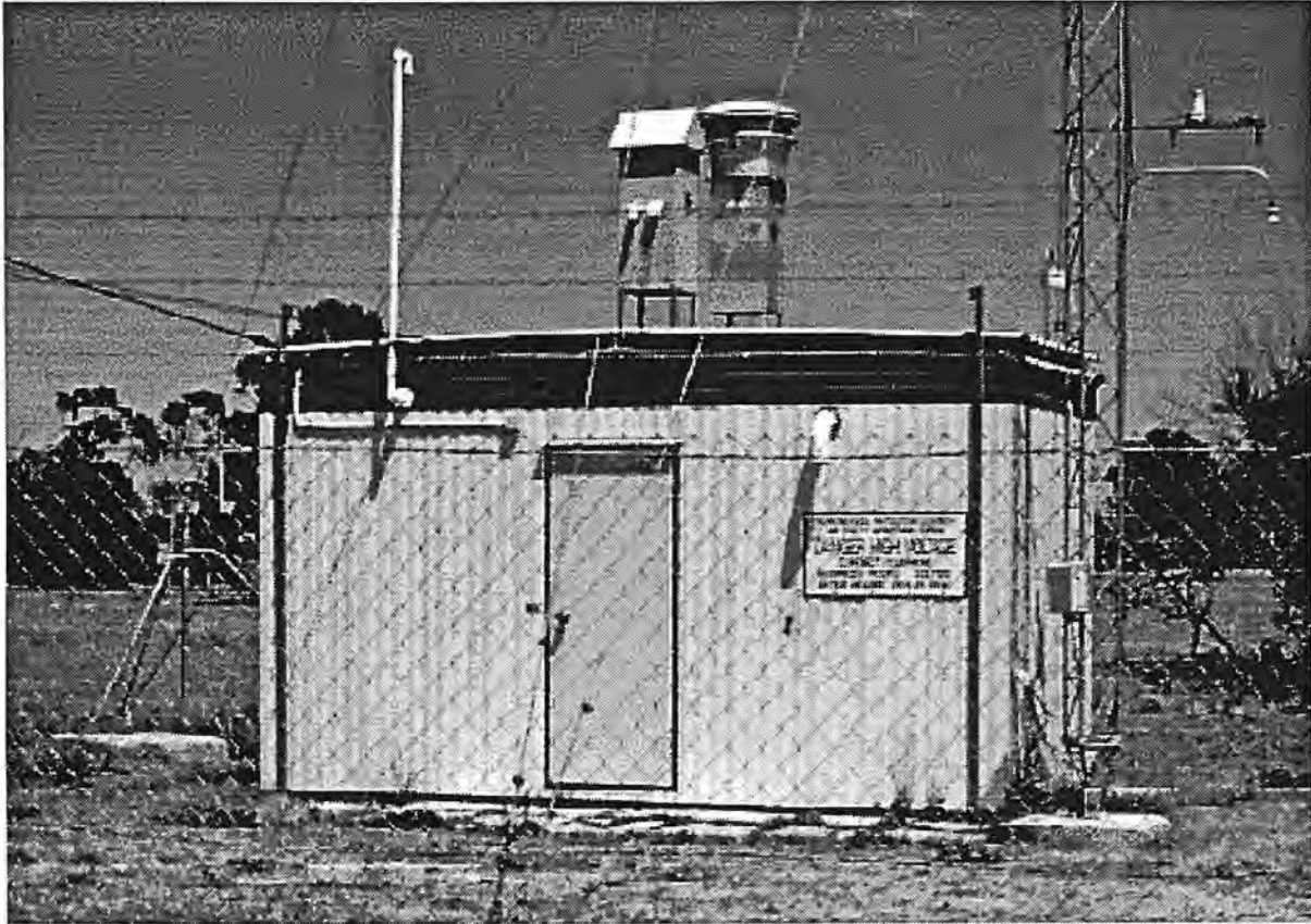
Figure 3.1 - Air quality monitoring shed at Caversham.
