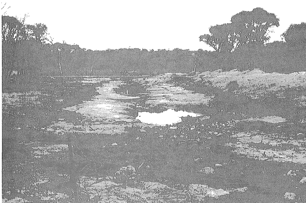
Eroded and excavated section of the Stoney Creek affected by salinisation. D2 Foreshore. Such drainage works can increase sediment and nutrient loss, if vegetation cover is sparse.
