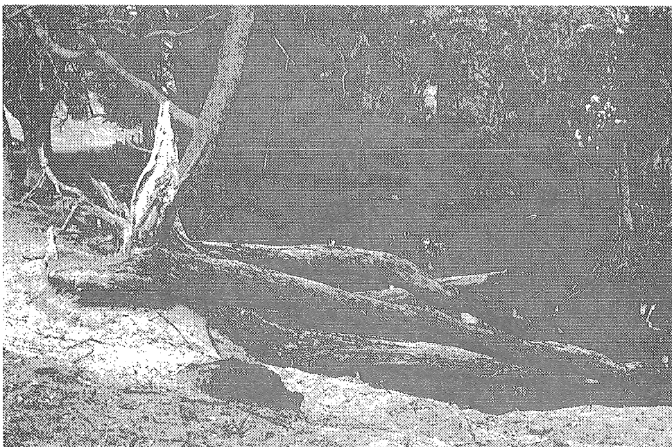
C Grade (left bank) and A Grade (right bank) along the Napier Creek, showing logs fallen into the waterway. These snags should not be removed, as they provide aquatic habitat. However, re-alignment at a 40-degree angle to the bank would minimise bank erosion.
