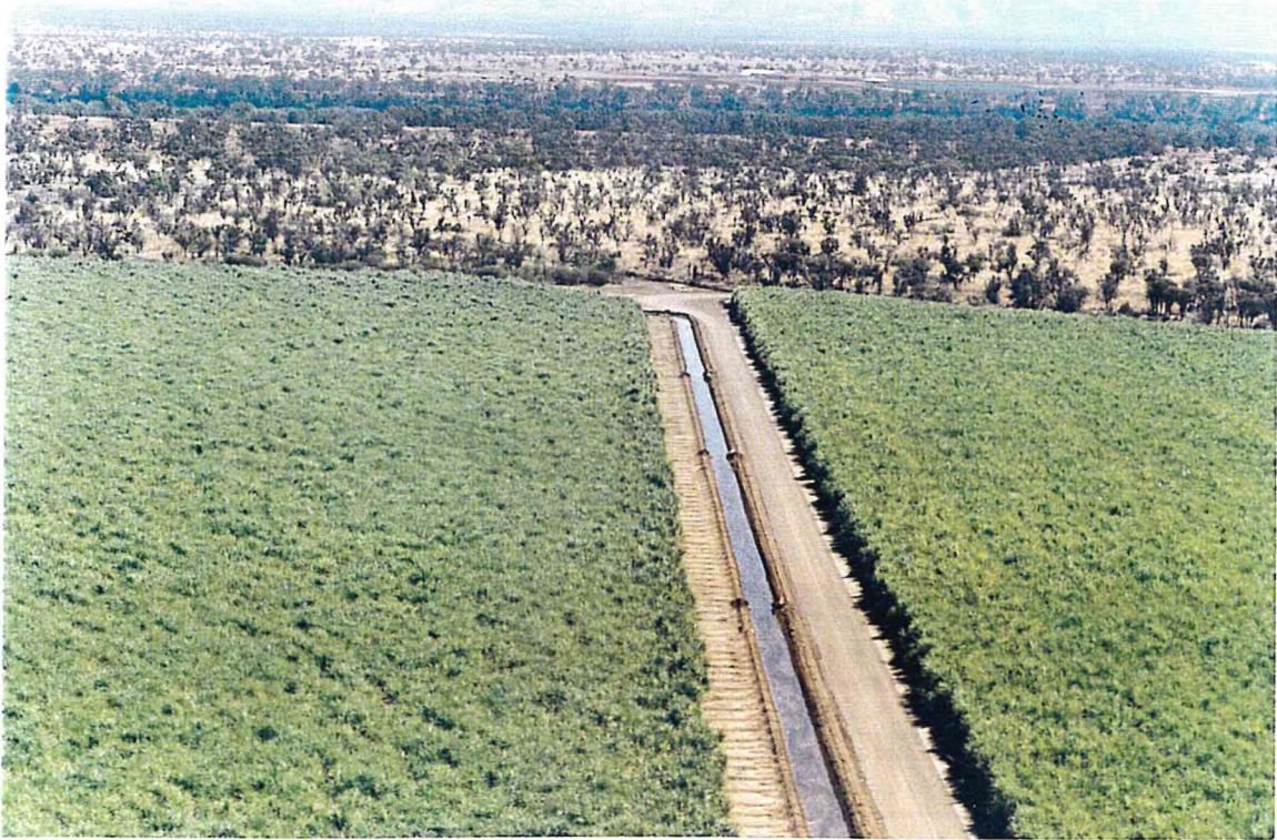
Figure 3-9 Irrigation channel in Ivanhoe Plains area of Ord Irrigation area
