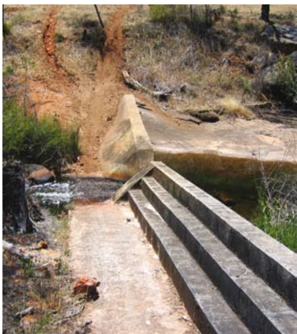
25 Ngangaguringuring gauging station and motorbike crossing (Ngangaguringuring gauging station-2)
