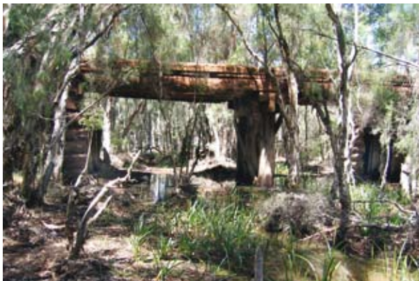
7 Firewood Road Bridge on the Helena River (Firewood Rd Bridge-2)
