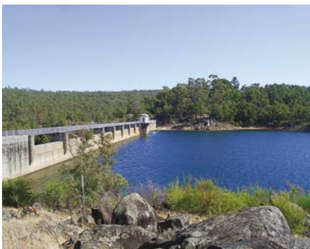
1 Mundaring Weir from the south (RIMG_0669)
