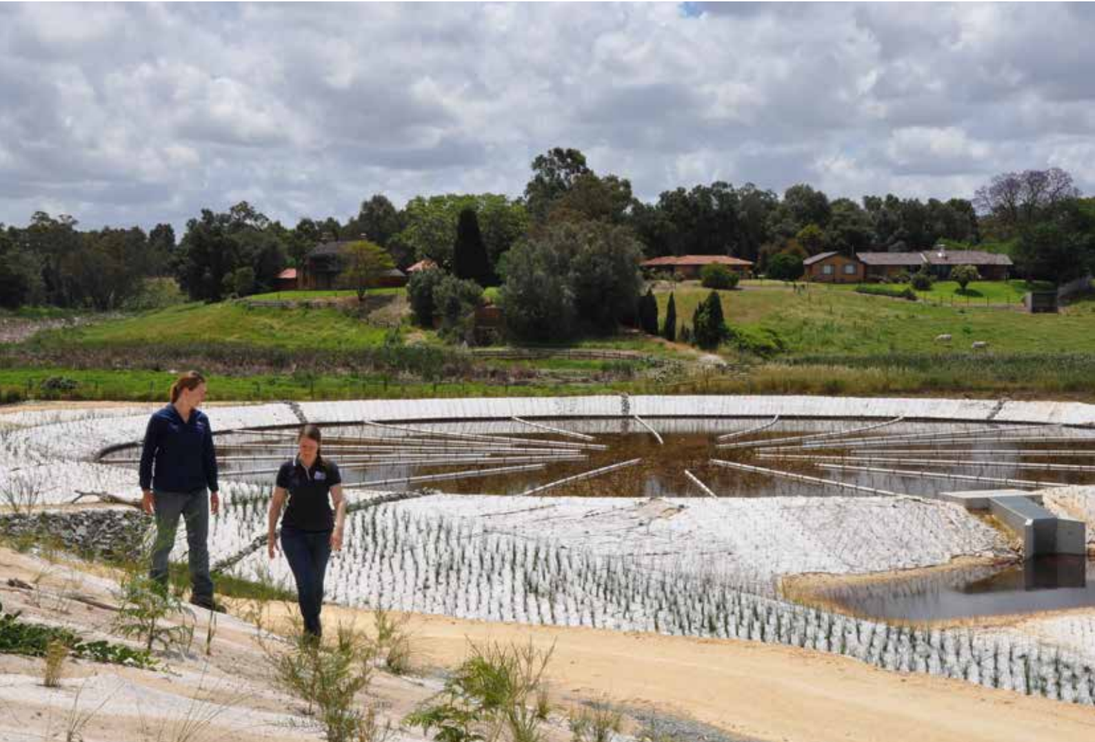
Kate Bushby and Christie Atkinson from the Swan River Trust at the Ellen Brook wetland. Stage one of the nutrient stripping wetland - which will reduce phosphorus and nitrogen reaching the Swan River - is now complete. Picture: Jennifer Eliot.
