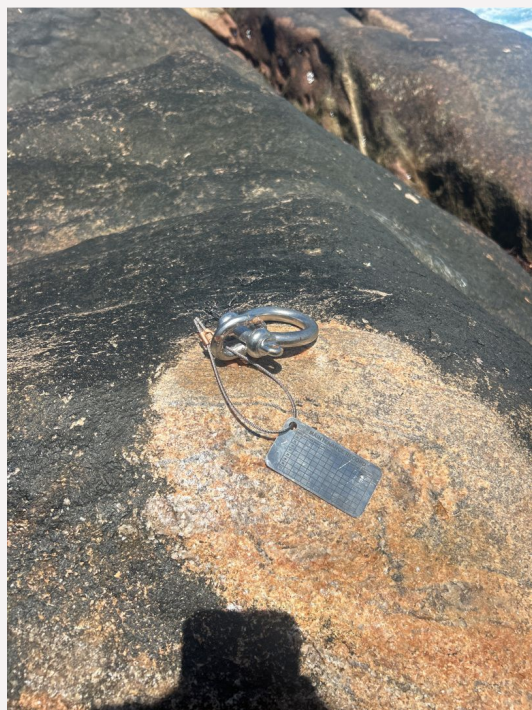
Images above: Marine Ranger Dean testing and tagging the rock anchors at Sugarloaf Rock.
