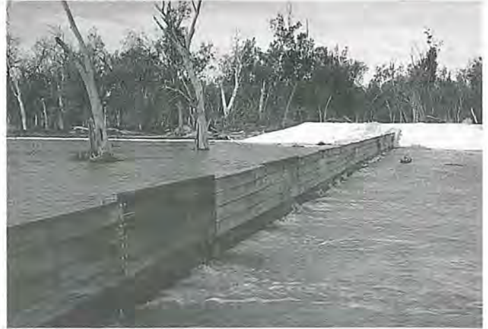
Separator gate shut, winter 1996, showing buildup and overflow into Toolibin Lake.
