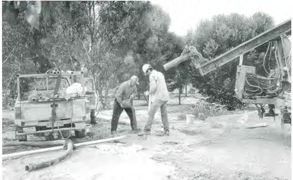
Bore program underway ...Agriculture Western Australia's Ben Whitfield (right) helps contractor Max Harris drill a bore at Dumbleyung as part of the Rural Towns Program.
