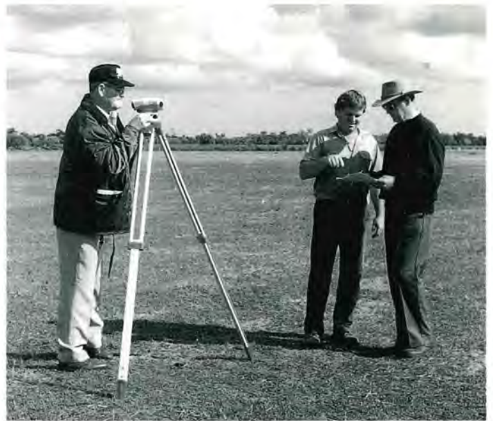
Farmer Trevor Massey (left) and John Adams from Challenger TAFE (right) receive instruction in levelling techniques from course presenter Nick Cox (AGWEST Bunbury) during "An introduction to the Planning and Pegging of Conservation Earthworks" at North Dandalup.
