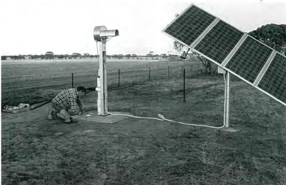
Ken Hodgkiss, Farm Manager for Toll, monitors a bore at 6.15am before the solar pump starts. The bore is 12 m deep, 125 mm casing and is fitted with a 8.5 cm poly piston pump to pump saline water into an evaporation basin. The pump yields 0.67 L/s under full sun.
