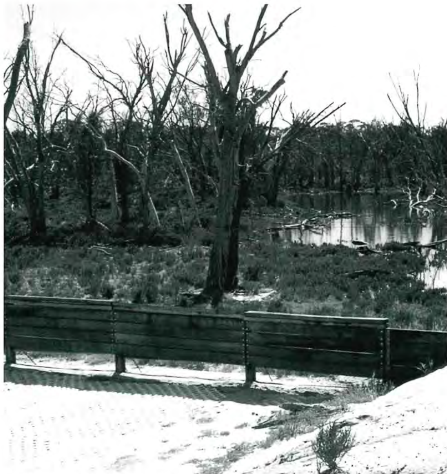
The Toolibin Lake Salinity Management System's range of engineering works helped win the salinity prize.
