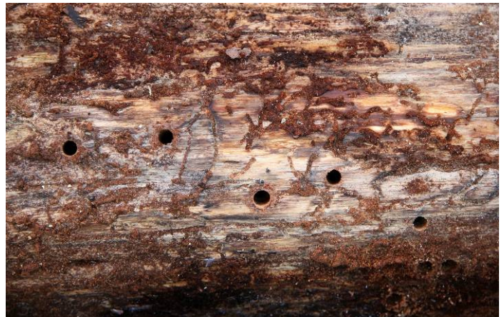
Sirex emergence holes surrounded by Ips and Hylastes galleries
