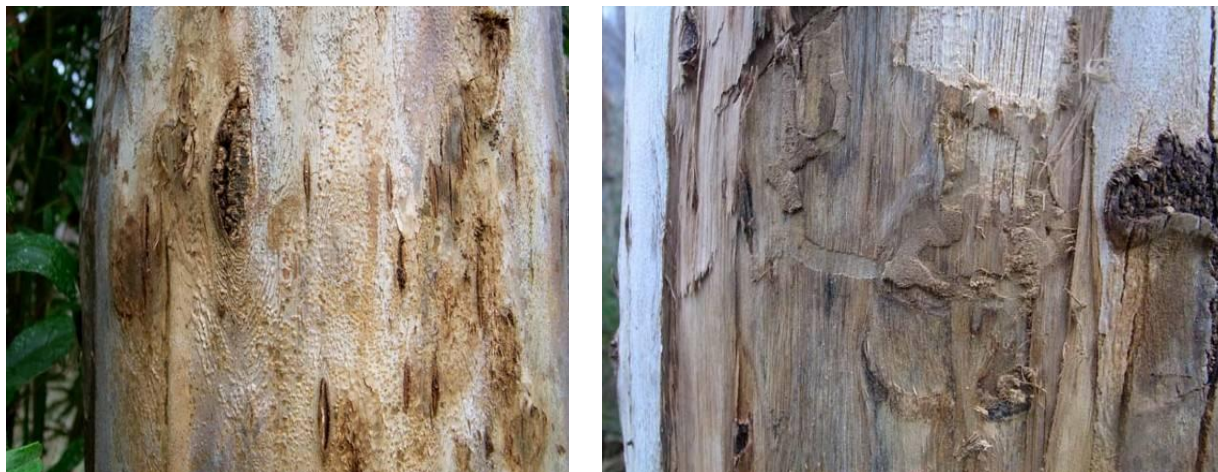
Figure 18: Holocryphia fruiting bodies and cankers (left) and borer galleries (right) in recently dead trees in a mid-rotation plantation in the north of the State.
