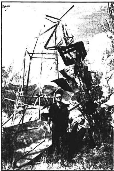
Left: One of the 350 water supplies damaged or destroyed by Cyclone Vance
