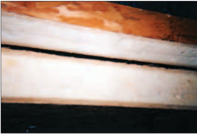
Figure 3—Cross section of a wall SIP.
