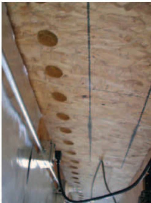
Figure 4—Incoming hot air holes (drilled through roof SIPs).
