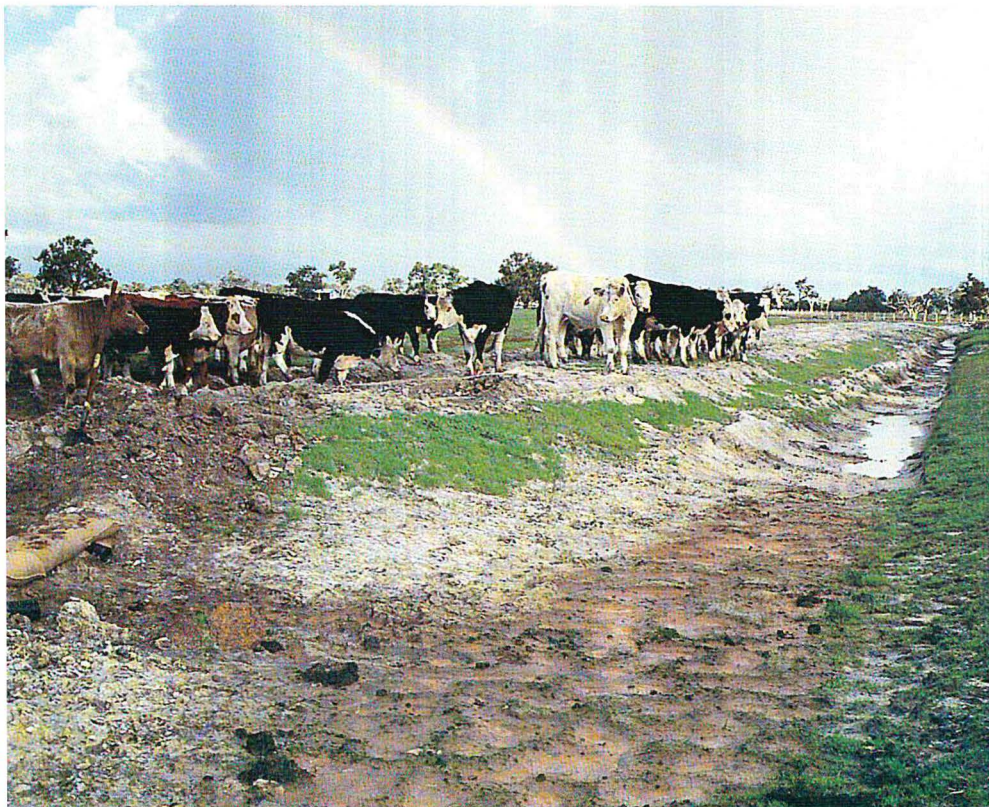
Drain bank damage of the Mealup Drain caused by stock trampling
