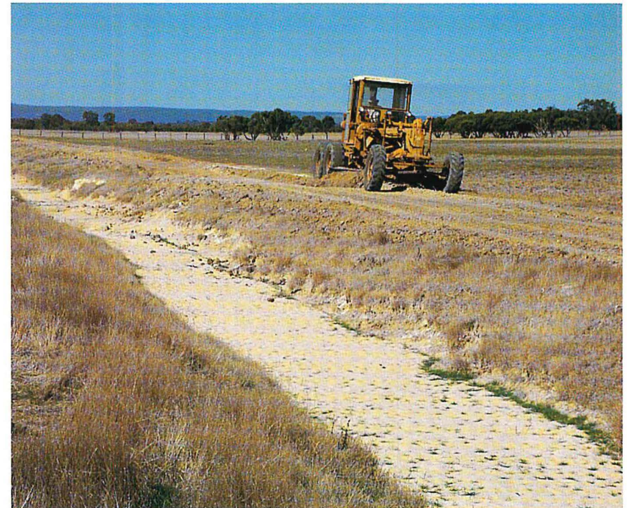
Grading the spoil bank of a drain in Kangaroo Creek area
