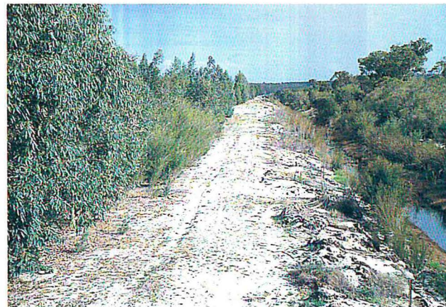
Meredith Drain streamlining, including the maintenance track
