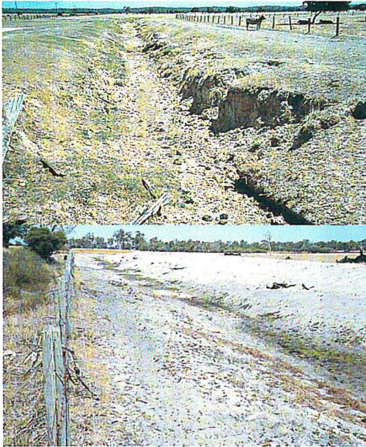
Two typical examples of the type of drain erosion
