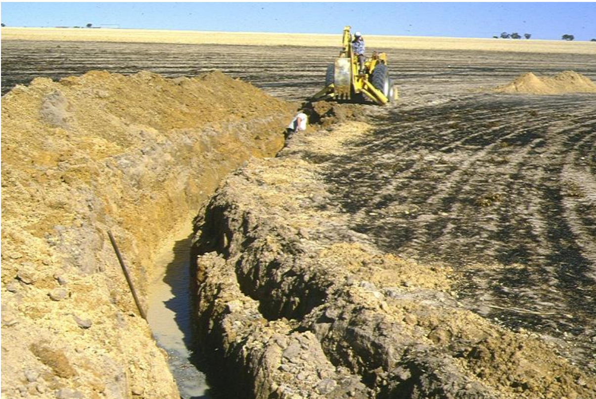
Constructing a deep drain on a sandpalm seep in the Wheatbelt.
