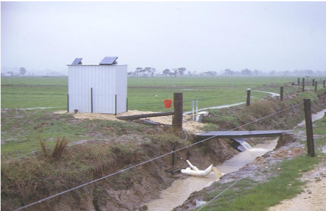
Surface and sub-surface drainage of irrigated pastures at Bengar.
