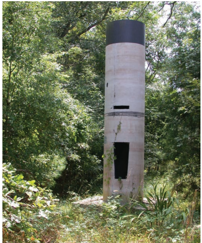
Figure 4—Concrete culvert tower roost installed on St. Catherine Creek National Wildlife Refuge. Seventy big-eared bats were observed using three of the structures in July 2007. (Photo by Alison McCartney)
