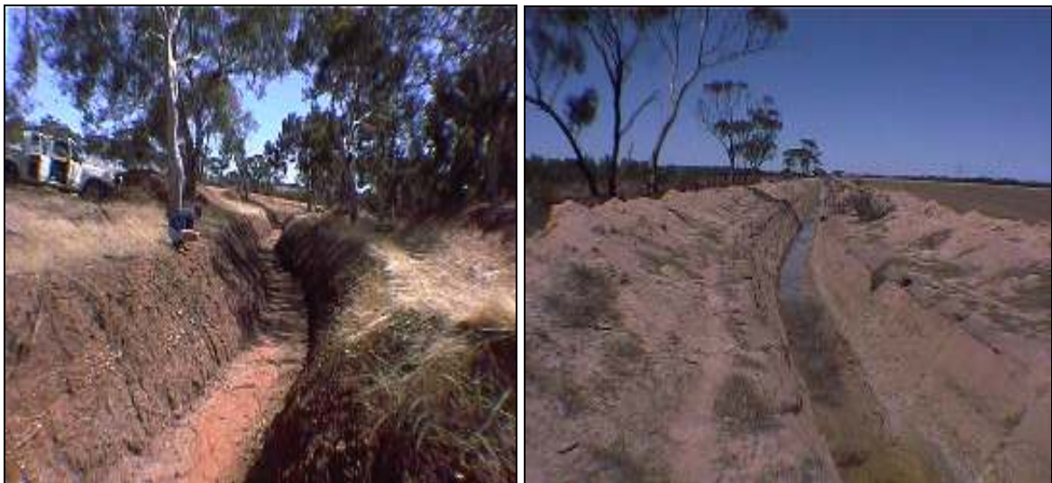
Figure 4.2.1 (a) Open deep surface drain in Watheroo and (b) Leveed deep surface drain in Kulin (Chandler 2002).
