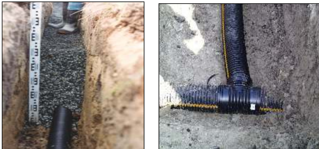
Figures 4.1.3 (a) PVC pipe drain backfilled with bluemetal; (b) A T-junction
