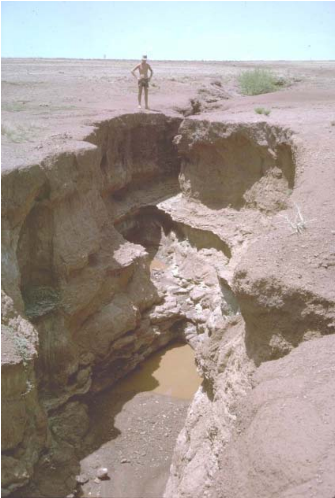
Photo 7. Gullies on the lower slopes of the Nelson land system were frequently incised many metres through the calcareous red soils and underlying soft shale and siltstone sediments. March 1964.
