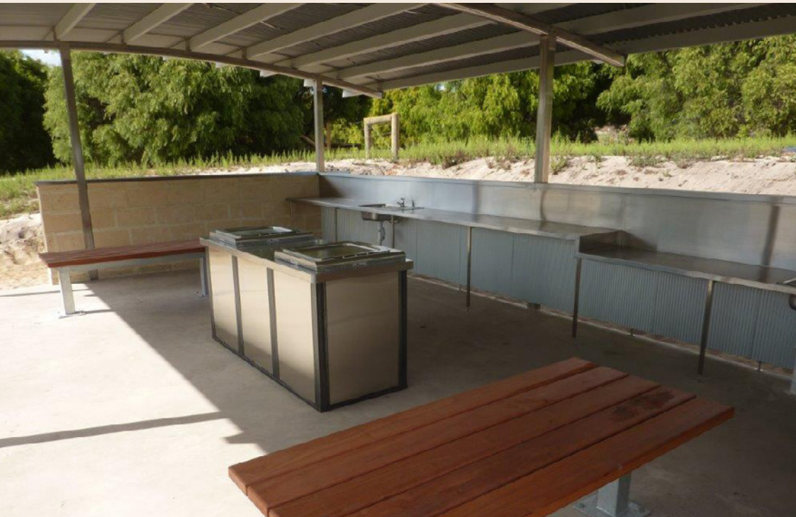
New shelter with barbecue facilities at Conto Campground. Photo – Glenn Willmott/Parks and Wildlife
