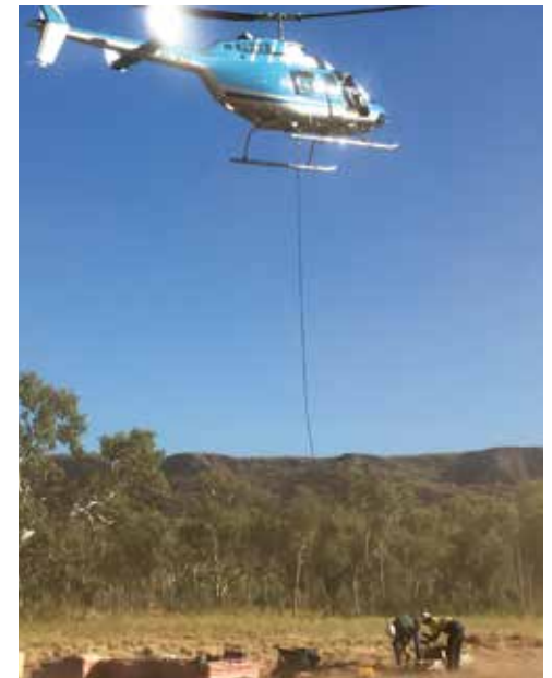
Transporting building materials by helicopter. Photos – Bill Dempsey/Parks and Wildlife
