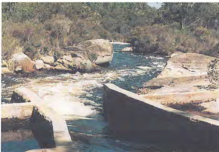
Collie River measuring flume downstream of Wellington Dam.
