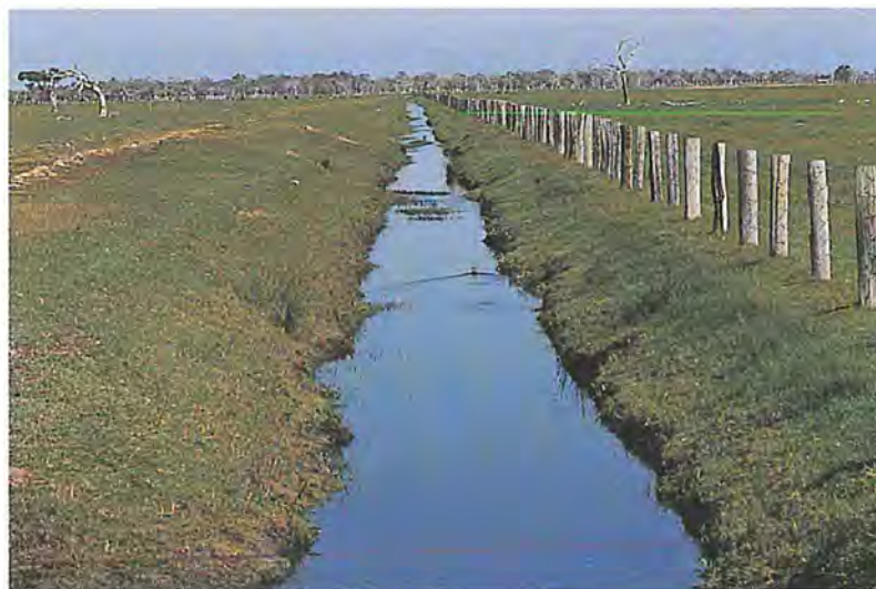
A drain in the Harvey River irrigation area.
