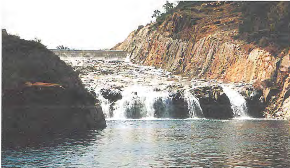
Harris Dam Spillway
