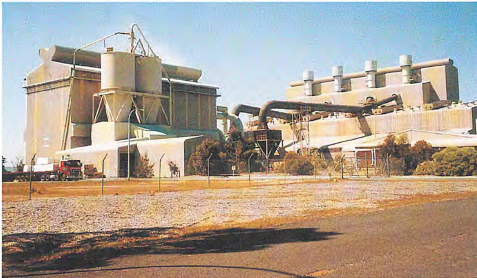
SCM Chemicals, Kemerton
