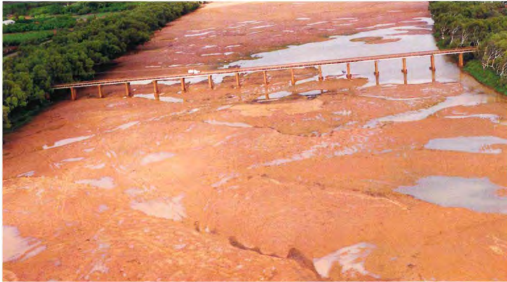
Aerial view of the Gascoyne River at Nine Mile Bridge
