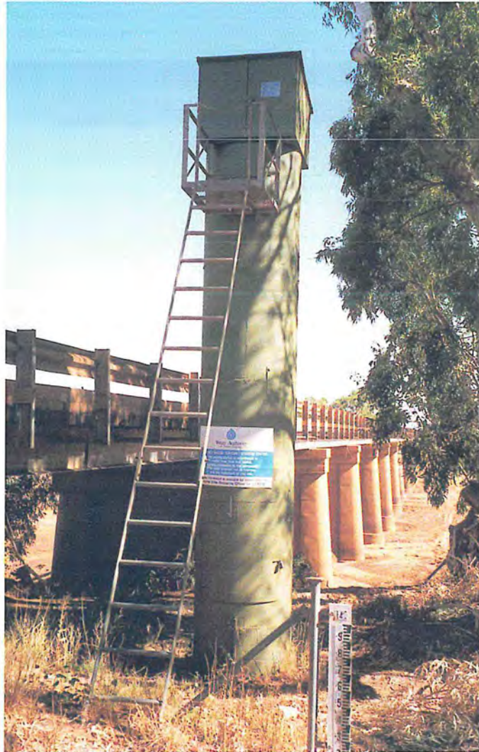
Nine Mile Bridge Gauging Station
