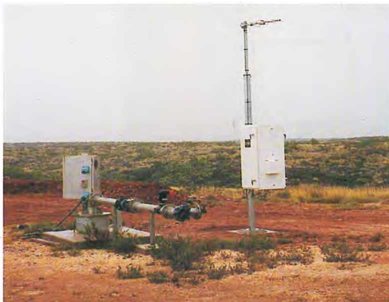
Groundwater production bore at Exmouth
