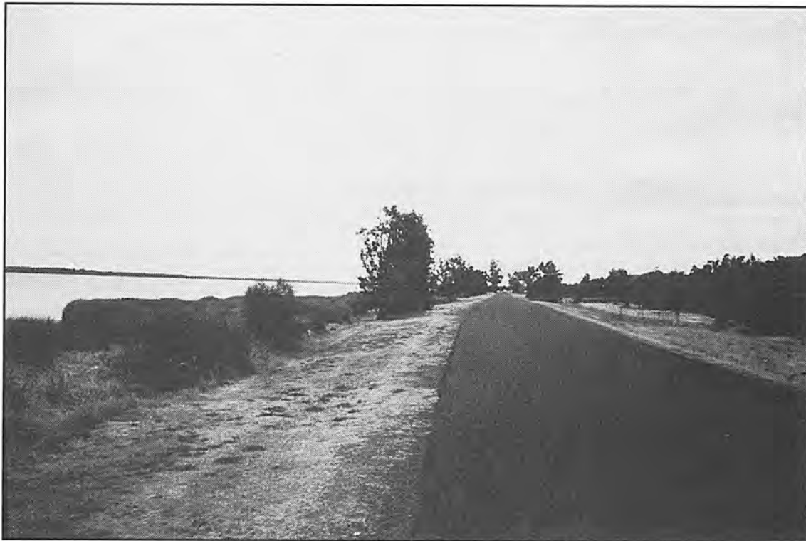
Plate 5: Cathedral Avenue has been widened at the southern end.
