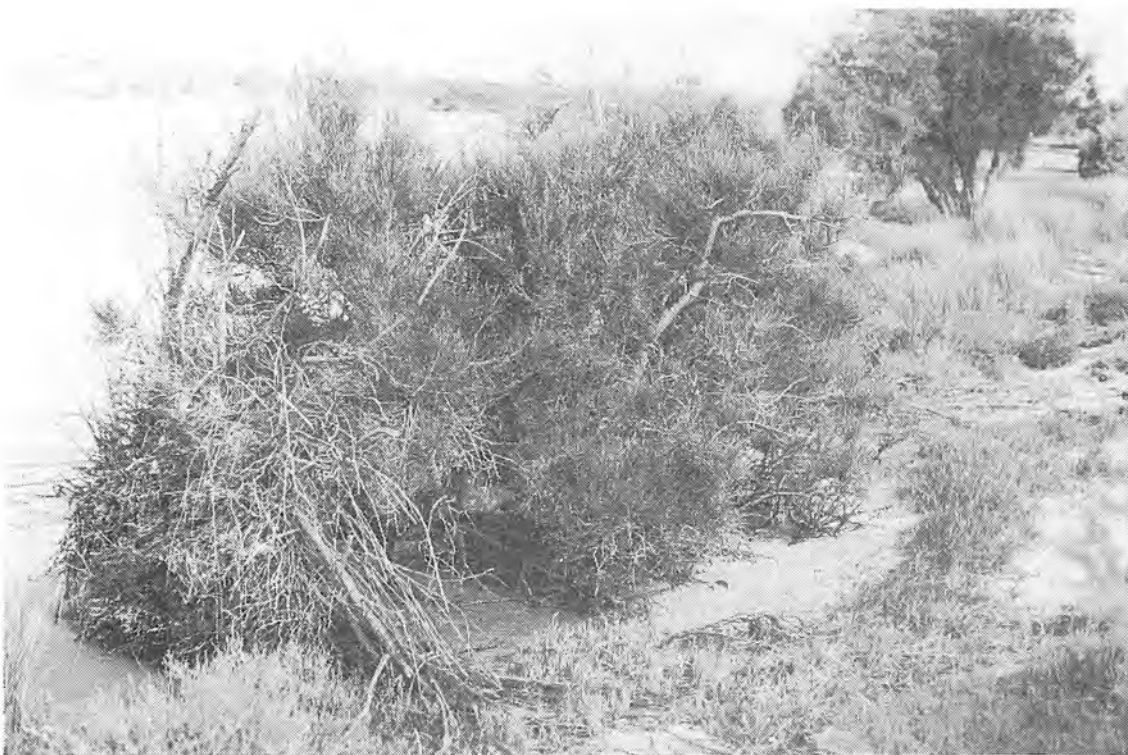
Photograph 2: Bar Island - erosion due to powerboat wash can result in the destabilisation of river banks
